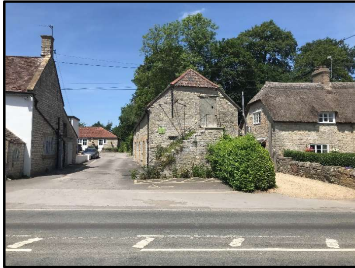
Landowner D photograph 1, notice on side of former stables.
